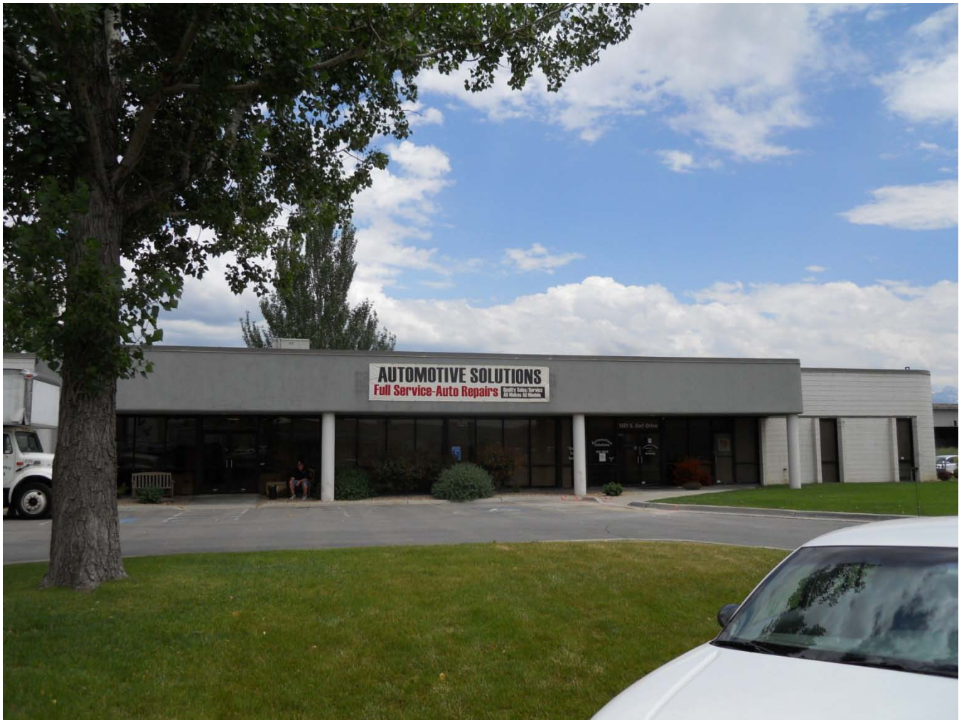
The existing south building on the property located at 1321 South Earl Drive.
